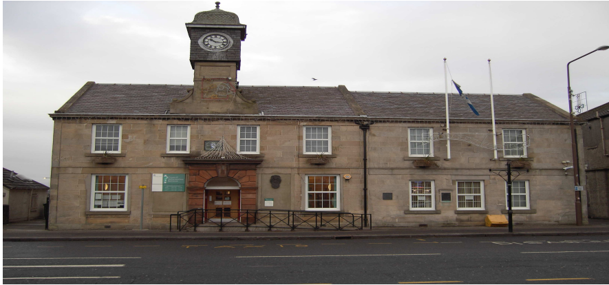
WHITBURN AREA OFFICE WINDOW REFURBISHMENT
